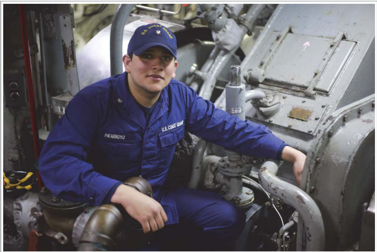
MK3 Felipe Patarroyo and other watchstanders responded quickly and accurate to a major lube oil leak.
